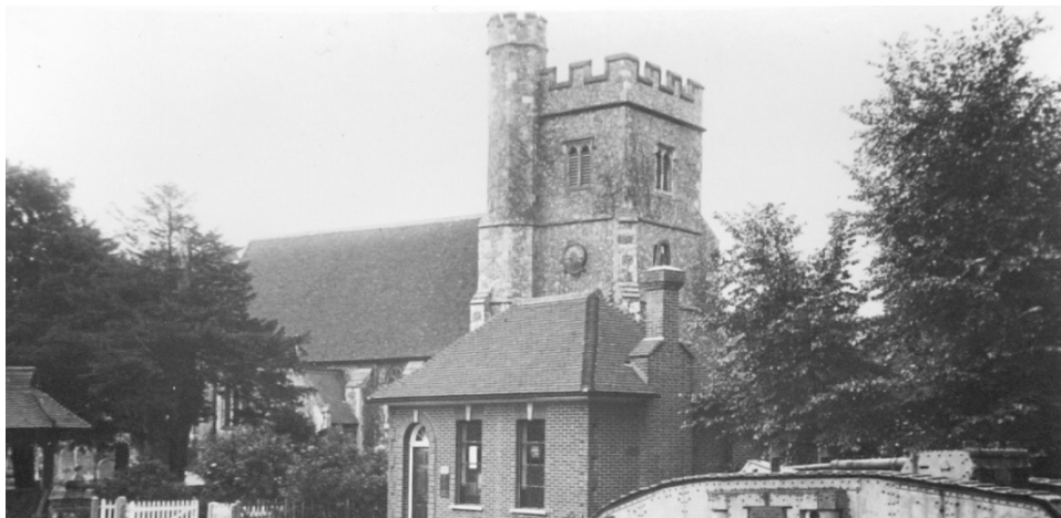
Farningham tank in the 1930s. The bank (then Martin's Bank, later Barclay's) was built in 1922. The tank was taken as war scrap in 1940. Sadly, the bank has closed this year and the building is up for sale.
